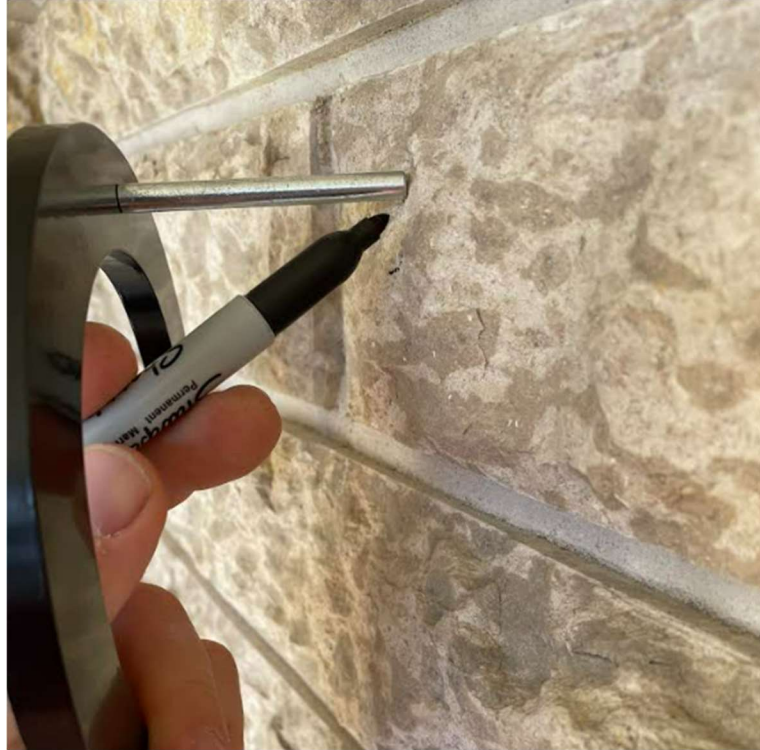
Figure 2: Mark the dowel location
