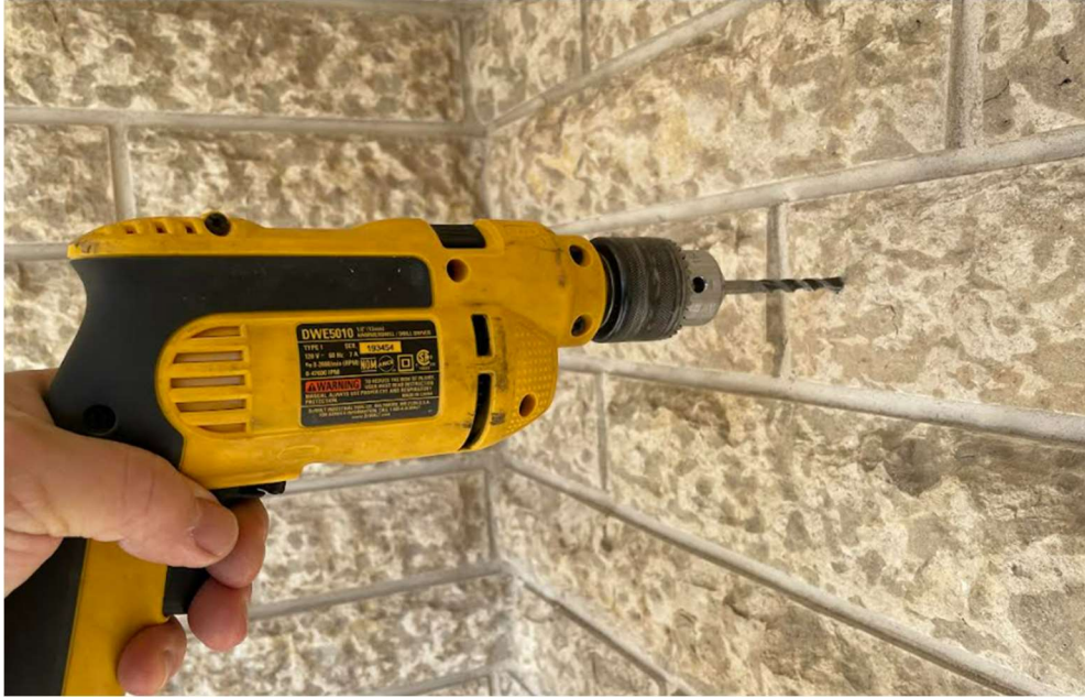
Figure 4: Drill the first hole
