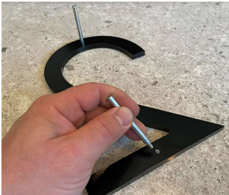
Figure 1: Install the dowels
